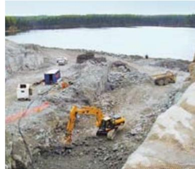
Under construction in Northwestern Ontario, the Lac Seul Generating Station will add 12.5 MW to OPG's hydroelectric capacity. The \$47 million project is expected to be finished in 2007. The station will use much of the water currently being spilled at the adjacent Ear Falls hydroelectric station, increasing the overall efficiency of the site.
